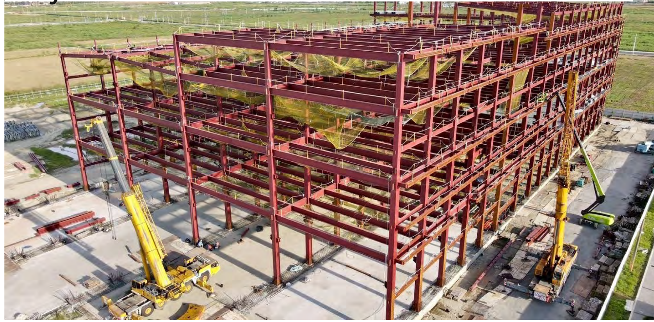
Structural Steel Works for Building A2 at Pingtung Chaozhou Railway station
